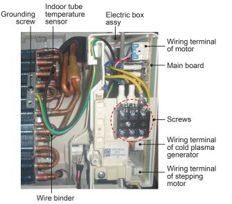
Rotate the electric box assy. Twist off the screws that are locking the wire clip and loosen the power cord. Remove the wiring terminal of power cord. Lift up the main board and take it off.
